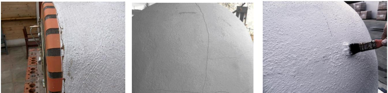
This is **absolutely normal** with all masonry wood fired ovens and not a serious problem which can be easily repaired with our **ULTRAFIRE SPECIAL REPAIR KIT** which is available from Euro Woodfired Ovens. Our **ULTRAFIRE SPECIAL REPAIR KIT** is a special waterproof concrete / plaster crack filler manufactured specifically for this purpose which can bridge cracks of up to 2.0mm.
